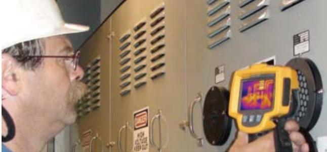
**Example of a thermographer using an IR window and wearing standard level of PPE required while operating energized electrical equipment in an enclosed and guarded condition.**
